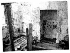
This large two storey flat and shop have been empty since the owner bought the property in 1994 (15 years ago). It is in a terrible state of repair and is no longer weathertight as most of the roof is now missing. This has resulted in the floor joists and boards becoming rotten. Parts of the floors are missing and the staircase is in a dangerous state. The whole property is completely derelict.
